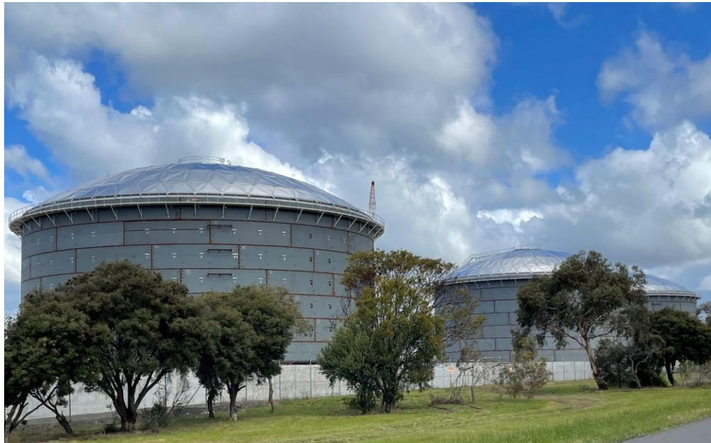
Construction of diesel strategic storage at Geelong – October 2023.
